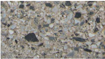
GROUND FACE SMOOTH, VISIBLE AGGREGATES
